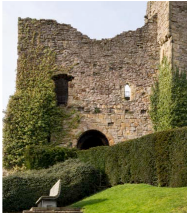
Figure 2 Exterior view of the east end of Scolland's Hall complex. The round-headed passageway sits below a line of postholes probably for a balcony, accessed by a door on the left. The latrine tower is on the right. DP184336 © Historic England Archive..
