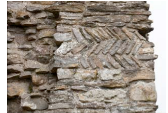
Figure 1 Detail of herringbone work from Scolland's Hall. DP233748 © Historic England Archive
